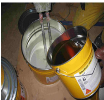
Mieszanie Sikafloor®-Comfort Adhesive i Sikafloor®-Comfort Porefiller.
